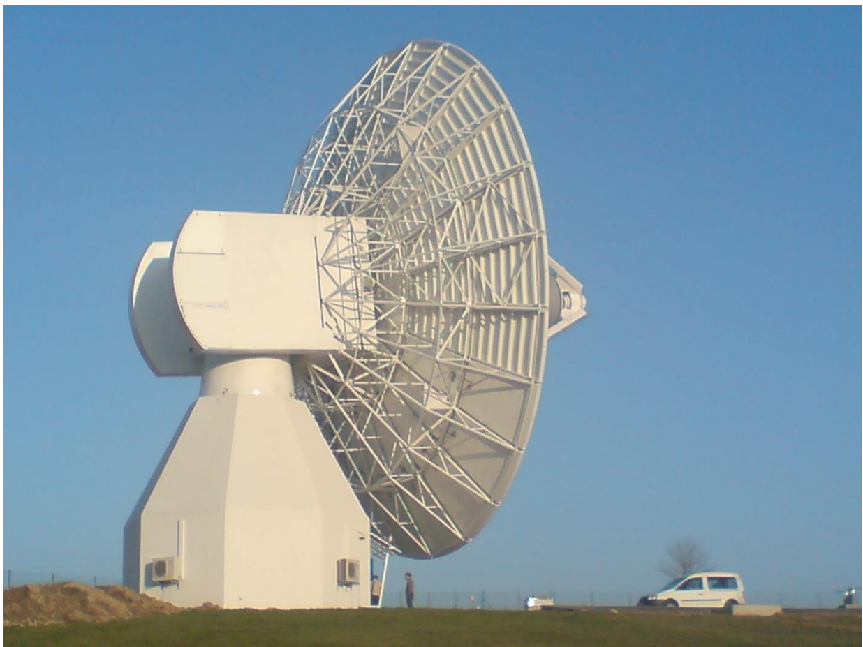
20 Meter Full Motion Antenna System
